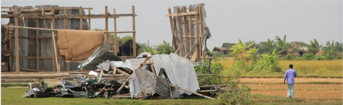
Collapsed house (in front) and partially destroyed mosque (in the back) due to the 10 October storm (Photo taken on 20-11-2012)
