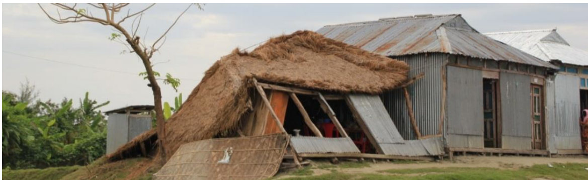
Shop damaged by the tropical storm of 10 October in Caring Char (photo taken on 20-11-2010)
