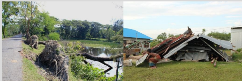
Uprooted trees on the way to Char Nangulia (taken on 19-11-2012) and a collapsed house in Noler Char (taken on 20-11-2012).
